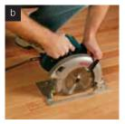
Using a circular saw or router, cut the board lengthwise to within 1/2" of the edges. For a glued board, make several cuts close together to separate the board into smaller sections.
