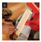
Trim the replacement board to the desired length, cutting excess length from the tongue end.
