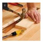
Remove nails or staples (this step does not apply to glued Engineered boards), then remove edges, taking care not to damage the adjacent boards.
