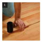
Install the board, using a rubber mallet and a wood block to place it in position.
