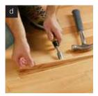
Using a wood chisel, remove the central part of the board first (between the side cuts).
