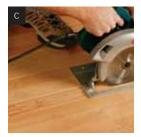
Make a diagonal cut down the center of the board from one end to the other of the cuts made in Step B. It may be necessary to make more than one cut if the board is glued in place.
