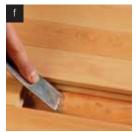
Remove the underlying construction paper or adhesive and clean any residue from the subfloor.
